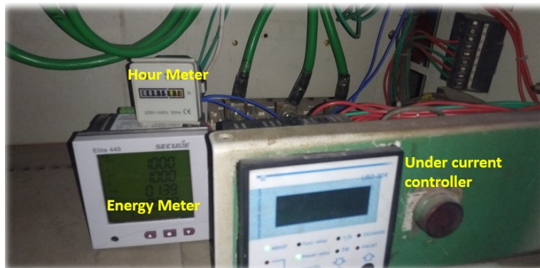
Figure 9. Experimental setup with energy meter, hour meter and underload detector.
